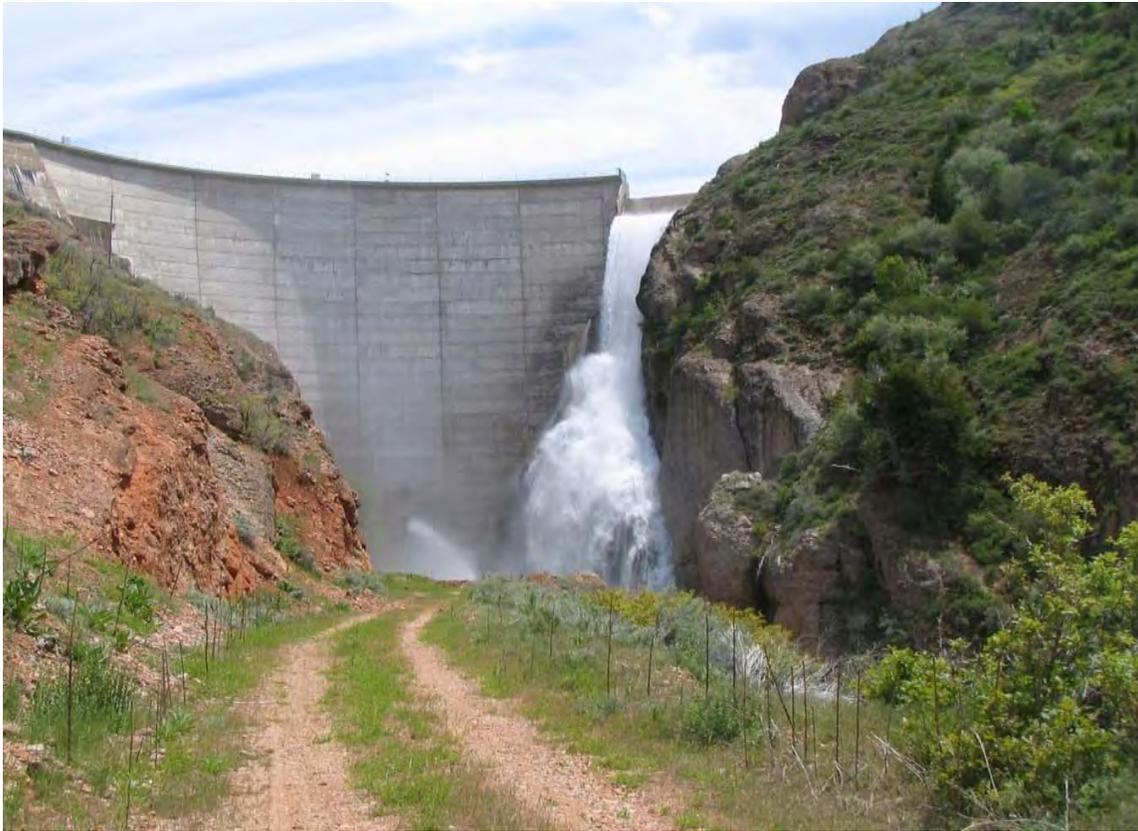
Figure 1.3.2-2 is a picture of East Canyon Dam spilling in June of 2008, (Provided by Nick Williams, USBR, 2008). Note the outlet discharge left bottom of spillway. Dissolved oxygen is reerated to saturation at the outlet. This image also helps visualize the steepness of the reservoir and why so much of the storage capacity resides in the upper elevations of the reservoir. The surface spillway skims the warmest water from the epilimnion in June, and may also export spring algal bloom biomass.
